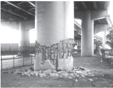
Figure 1– Crushed RC column under seismic loads
